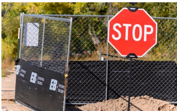
6. Equipment/roadway paths must be properly marked with tape or barricades to delineate between roadway and personnel areas.
