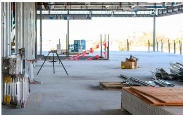
5. In general, jobsites should be tidy/organized, so keep an eye out for potential trip/fall hazards.
